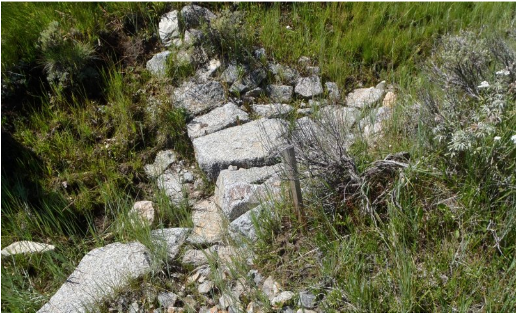
Figure 10. New rock work at headcut
